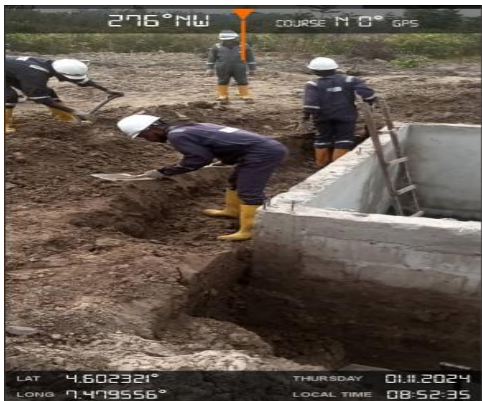
Plate 2: Excavation round the sump for plastering
