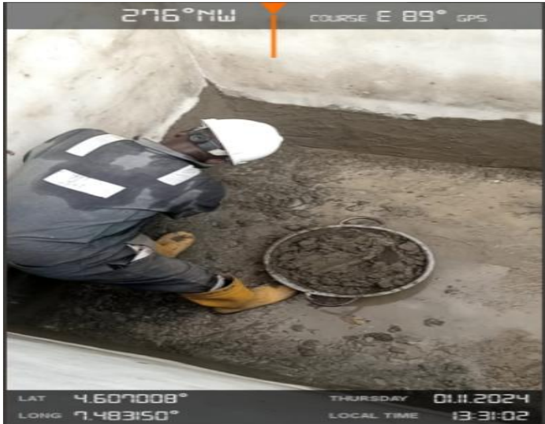
Plate 3: Plastering inside the sump
