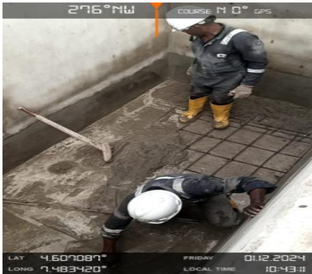
Plate 4: Flooring of the sump
