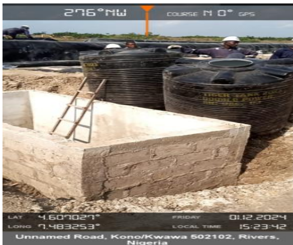
Plate 6: Gee Pee tank going into the sump
